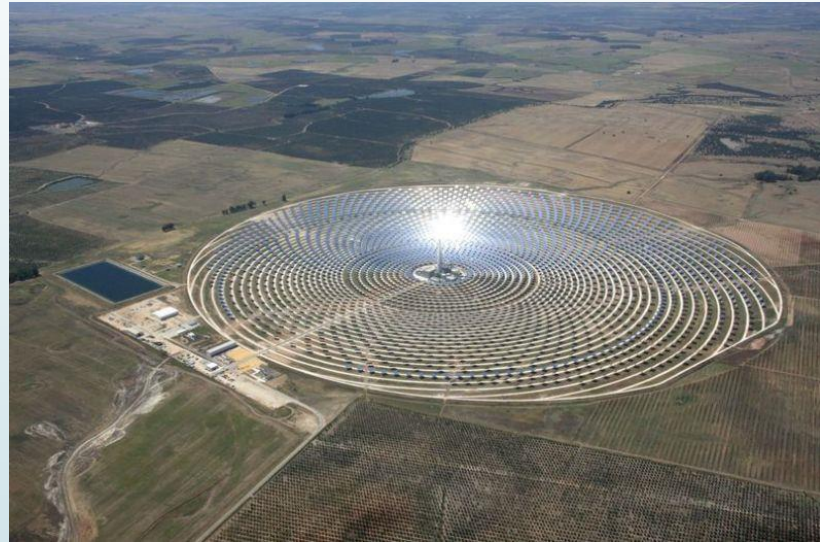
Gemasolar plant in Spain, Andalucía
