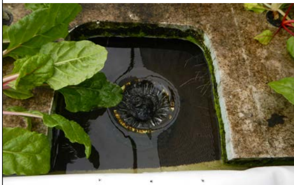
FIGURE 9.14 Stand pipe in a deep water culture canal maintaining the water column height
