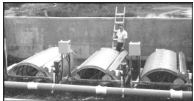
3 models 1607-2H with flow capacity = 16000 gpm
