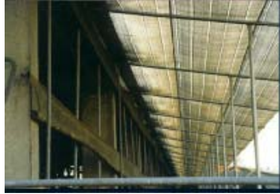
Figure 11b. Improved side curtains
