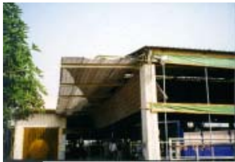
Figure 12b. West side of the dairy barn after renovation (view 1)
