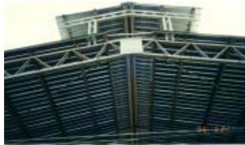
Figure 12a. West side of the dairy barn before renovation
