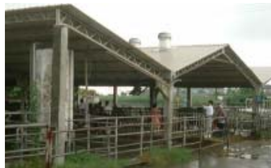
Figure 14b. Wind driven rotating roof vent.
