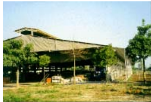
Figure 12c. West side of the dairy barn after renovation (view 2)
