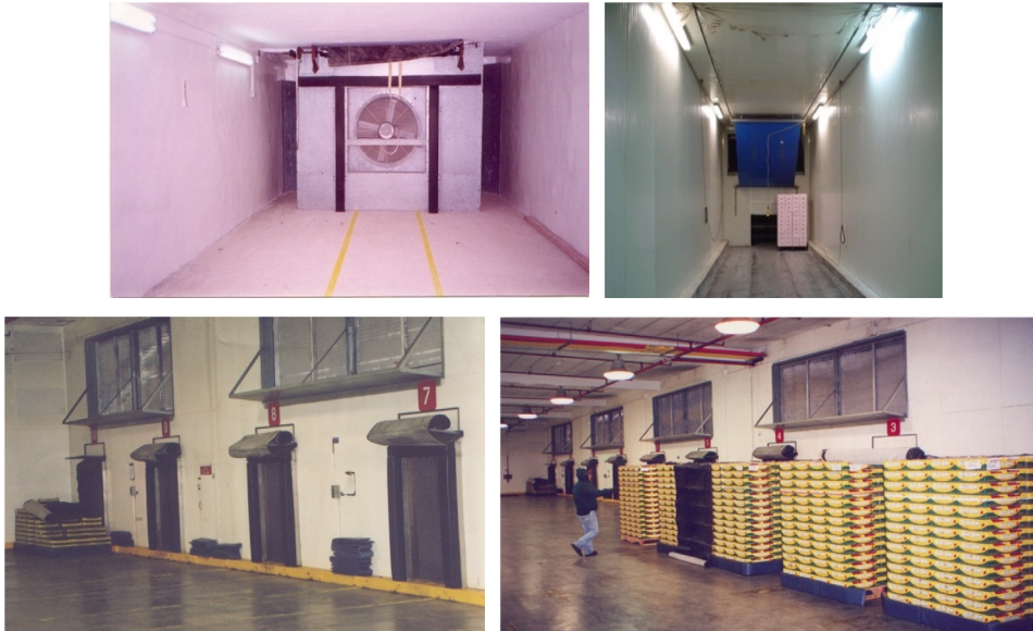
FIG. 6.5 Forced air precooling system.
