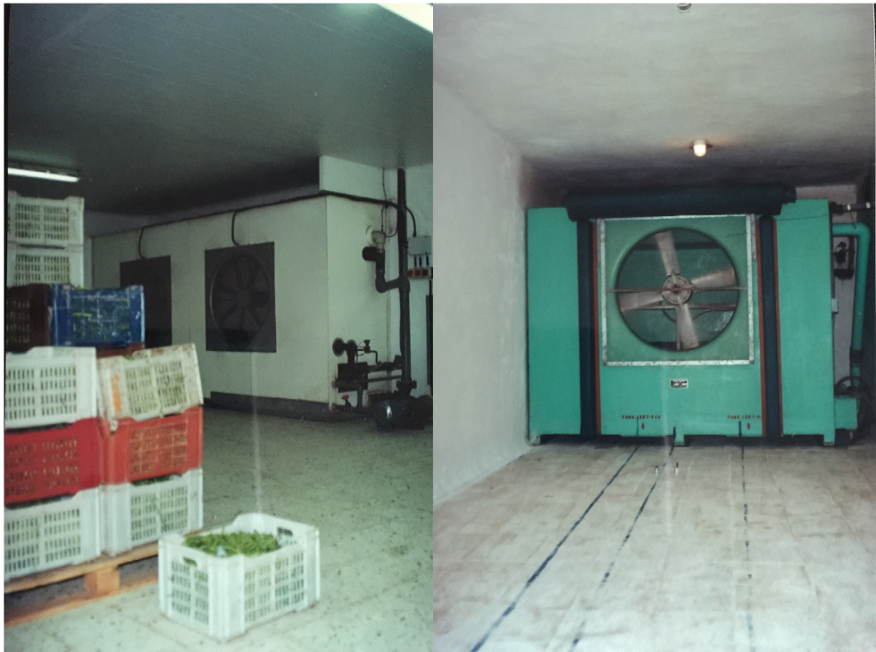
FIG. 6.9 Ice Bank (wetted coil).
