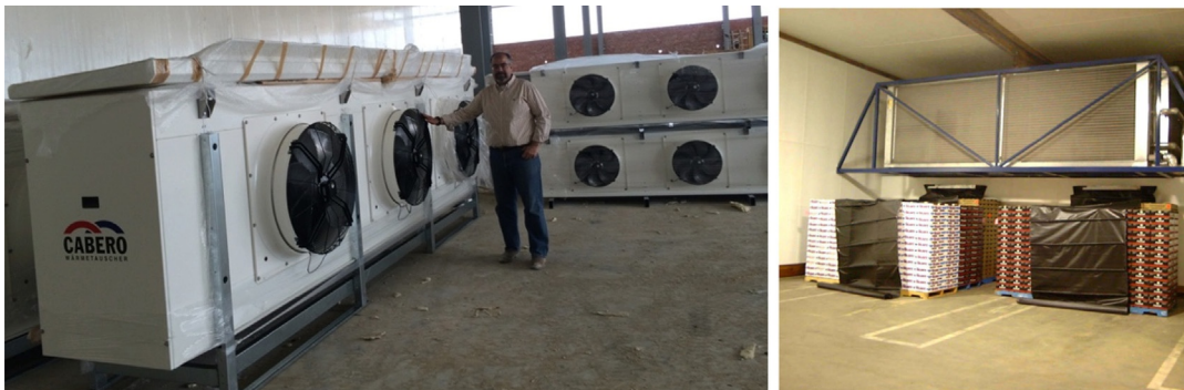
FIG. 6.10 Typical evaporative coil for the dry coil high humidity system with large surface area.
