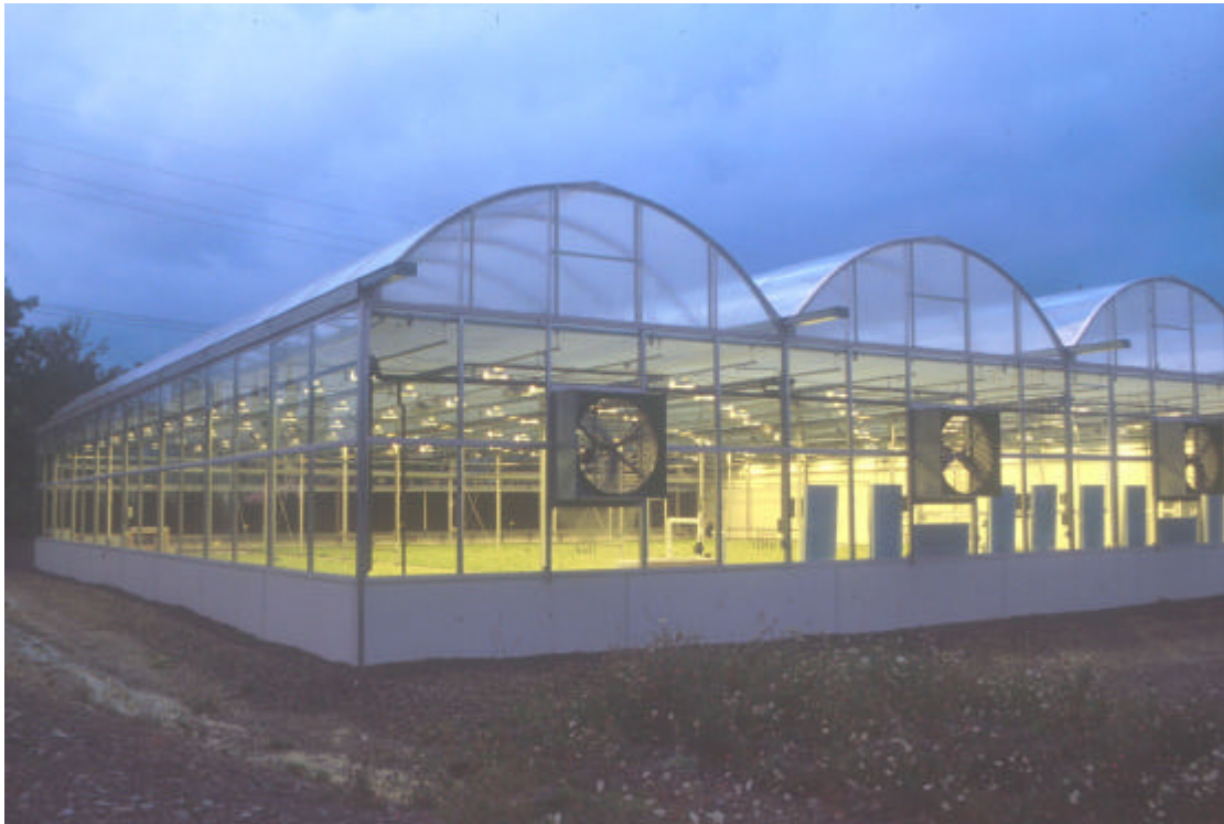
Photo 1. Outside view of the 750 m 2 hydroponic lettuce demonstration greenhouse in Ithaca, NY, USA. This facility produces 945 heads of lettuce every day of the year using the floating hydroponics system. The total production cycle is 35 days; 11 days in an environment controlled growth room and 24 days in the greenhouse. At 150 g per head (fresh mass), this greenhouse facility has the potential to produce just over 51,000 kg of edible biomass annually (68 kg·m -2 ·yr -1 ).
