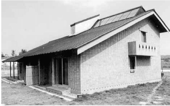
Fig. 2. Southeastern view of experimental house.
