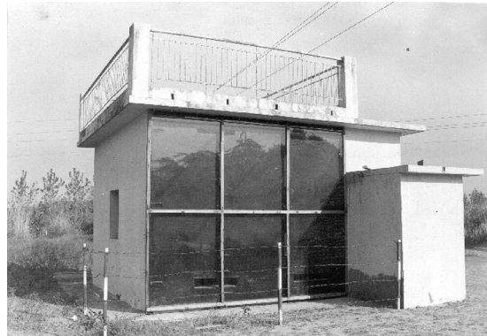
Fig. 9. Photograph showing overall view of the passive model 2 building.
