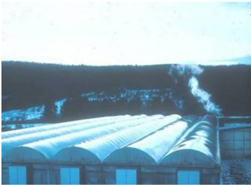
Gutter-connected steel-frame greenhouses with double-poly roofs
