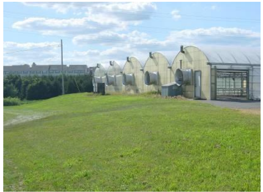
Gutter-connected steel-frame greenhouses with double-poly roofs
