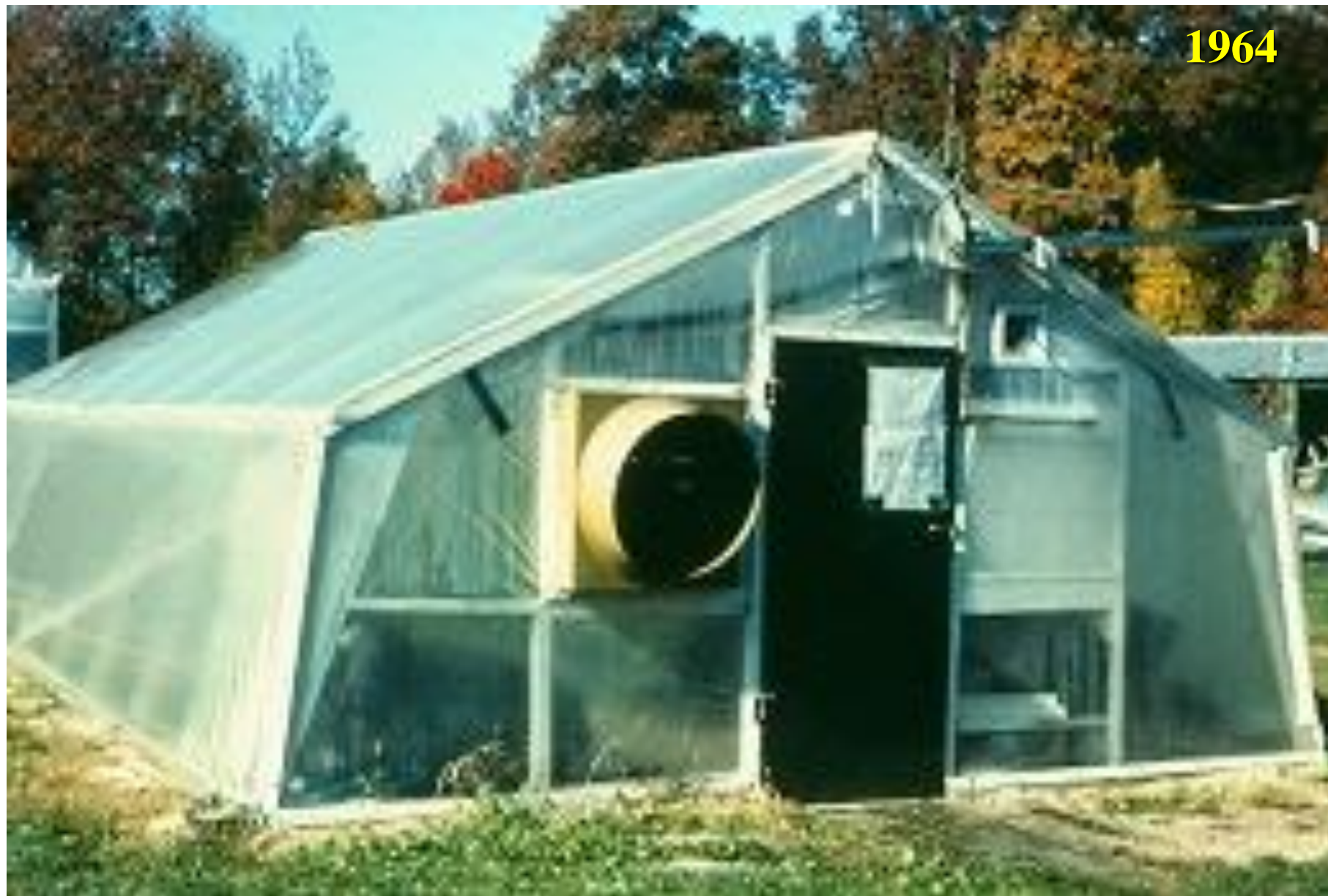
First greenhouse with double poly
