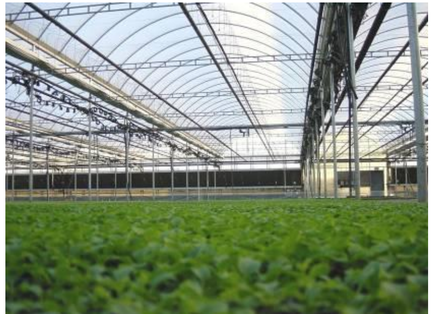
Gutter-connected steel-frame greenhouses with double-poly roofs
