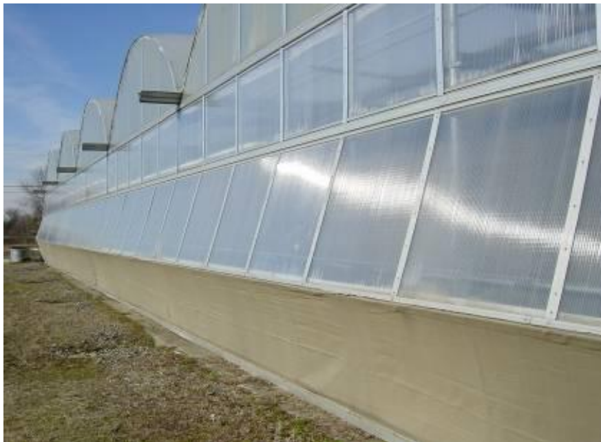
Gutter-connected steel-frame greenhouses with double-poly roofs
