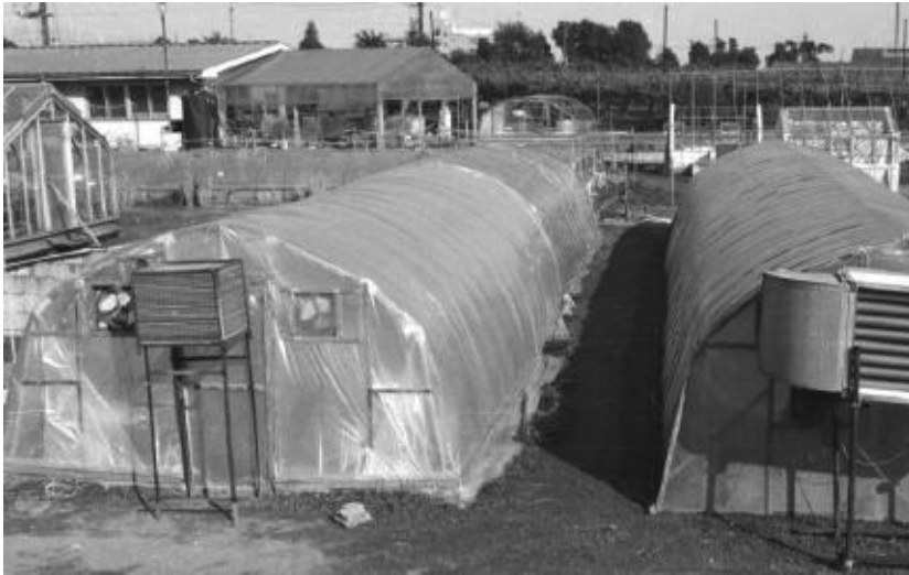
Typhoon attacked greenhouses, but no damage on double-poly
